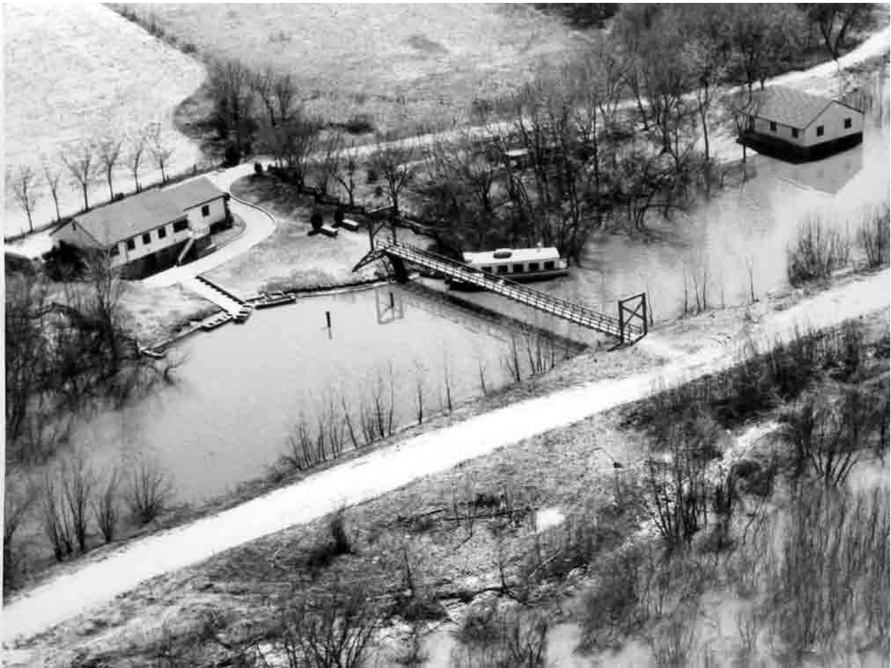
During the depression years of the 1930s, the federal government established work programs that made possible a variety of construction projects. The Survey made use of that opportunity to construct a building to house the Havana Station. The frame structure was completed in 1940, a mile or so from the site on Quiver Lake where Forbes had established the station in 1894.
